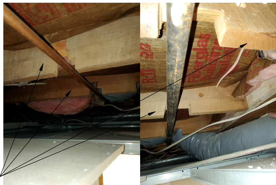
D4 EXISTING JOISTS TO BE REPLACED SCALE: 3/4" = 1'-0"
